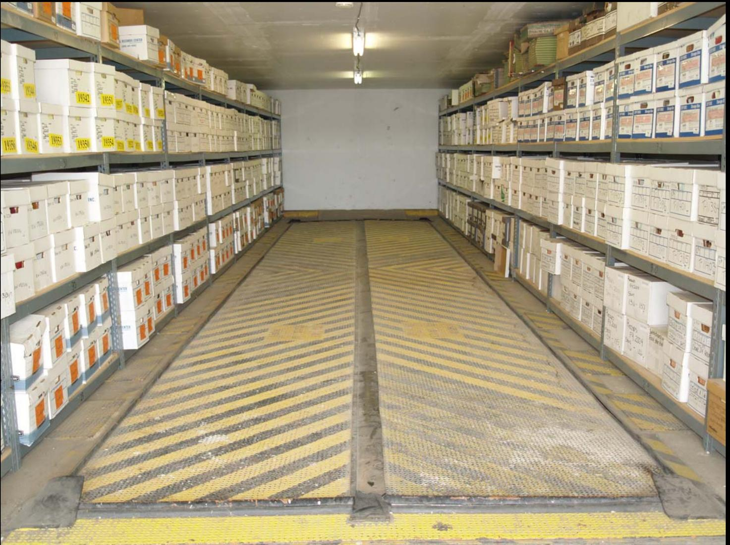
**The uniqueness of the NIKE missile sites were their underground storage of the missiles. This picture is of the top of the elevator. The elevators are about 50 feet long and ten feet wide and were used to bring the missiles to the surface so they could be launched. Our site has three missile bays.**
