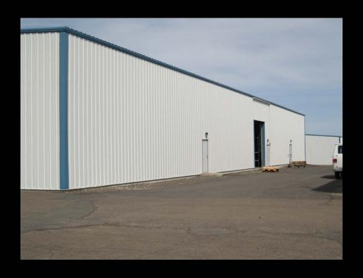
Our new building style is shown above. They are all steel construction and are 104' by 171'. This design allows us to store your records on properly installed steel shelving. Maximizing the amount we store per building but protecting the integrity of the boxes your records are stored in.
