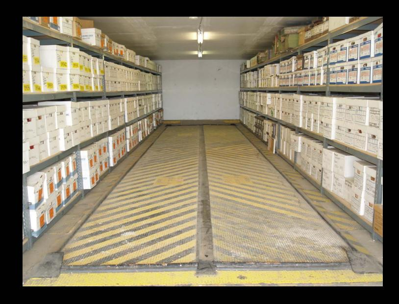
The uniqueness of the NIKE missile sites were their underground storage of the missiles. This picture is of the top of the elevator. The elevators are about 50 feet long and ten feet wide and were used to bring the missiles to the surface so they could be launched. Our site has three missile bays.
